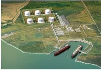
* Sabine Pass LNG, L.P. Cheniere Energy Partners, L.P. Cheniere Energy, Inc. 91%
