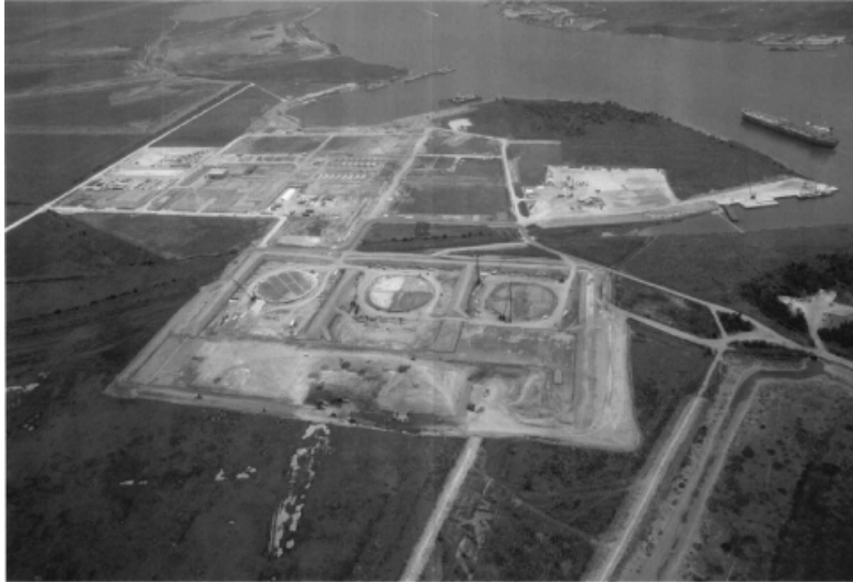
Aerial View from the North
