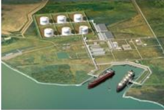
* Sabine Pass LNG, L.P. Cheniere Energy Partners, L.P. Cheniere Energy, Inc. 91%
