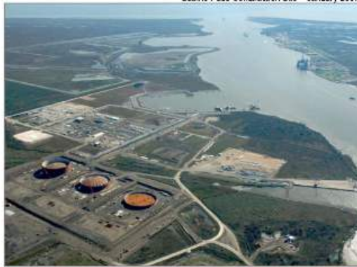
Sabine Pass Construction Site – January 2007
