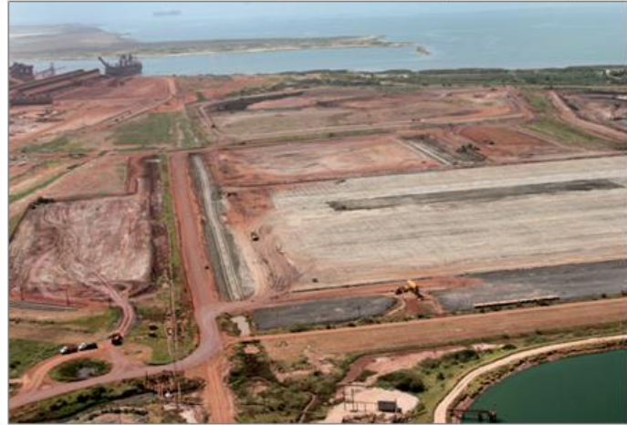
Corpus Christi Site Preparation
