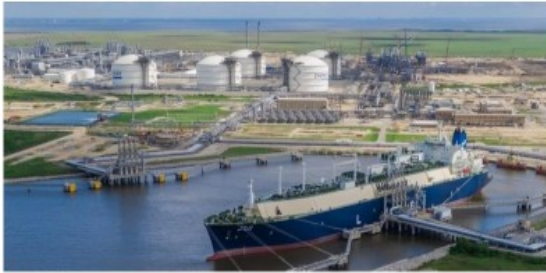
Sabine Pass Liquefaction Project (Louisiana)
