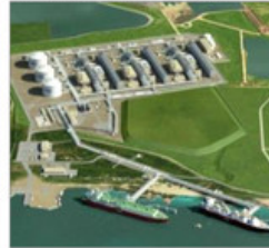
SPAs with CCL First LNG Expected 2018
