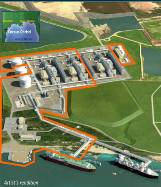
Artist's rendition Design production capacity is expected to be ~4.5 MTPA per train, using ConocoPhillips' Optimized Cascade® Process.
