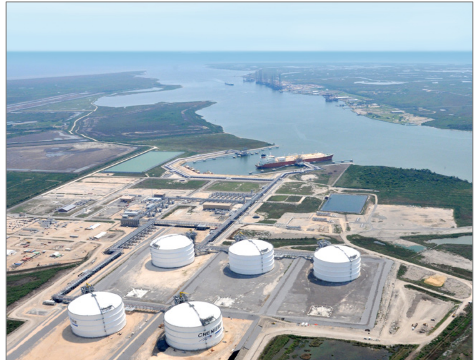
Aerial view of Sabine Pass LNG Terminal
