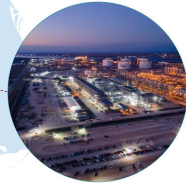
Sabine Pass Liquefaction ~30 mtpa Total Production Capacity
